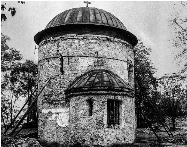
Il. 7.2.21 Rotunda podparta stemplami, widok od wschodu, 1942 (fot. A. Müller) ¶ Rotunda shored up with props, view from the E, 1942 (photo: A. Müller)
