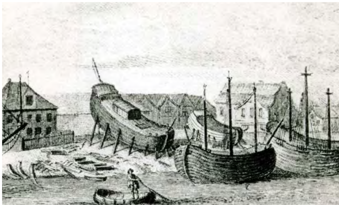
Fig. 8. Part of a drawing by F. A. Lohrmann from 1770 showing the Brabant shipyard in Gdańsk: on the water – a galliot being fitted out, and in the background – a cat in the course of construction (Polish Academy of Sciences Library, Gdańsk).
