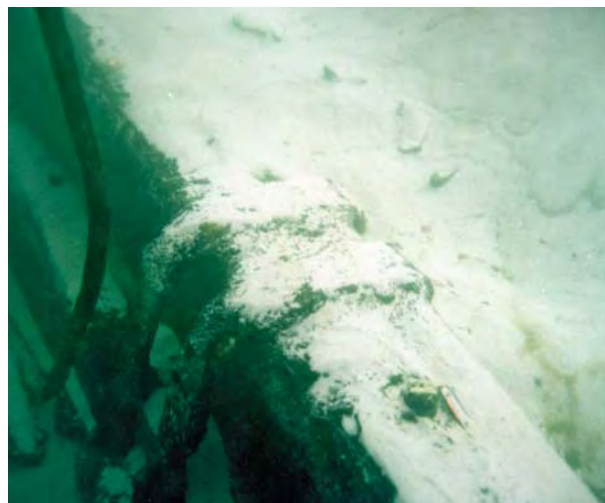
Fig. 7. Metal reinforcement of the scarf joining the timbers of the keelson (photo by W. Ossowski).
